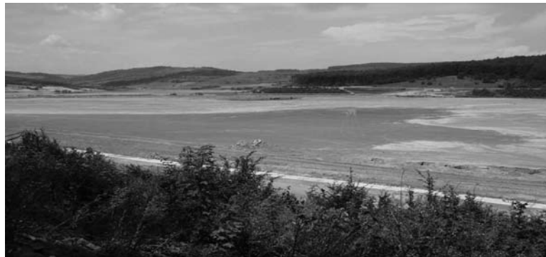
Fig. no.3. Wet the surface of deposit - effective solution to protect the winnow
