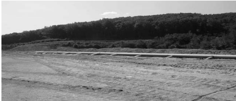
Fig. no.4. Pipe with holes raw water wetting of the surface storage
