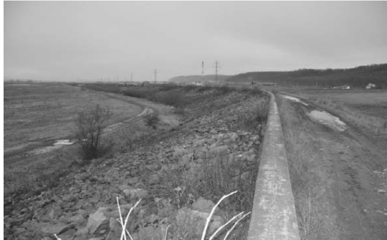
Photo no.4 Rockfill laid-down on the protection dam made on Jiu river upstream Rovinari mining coal perimeter
