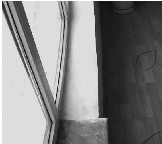
Fig.6. Condensation at the inferior edge of the window
