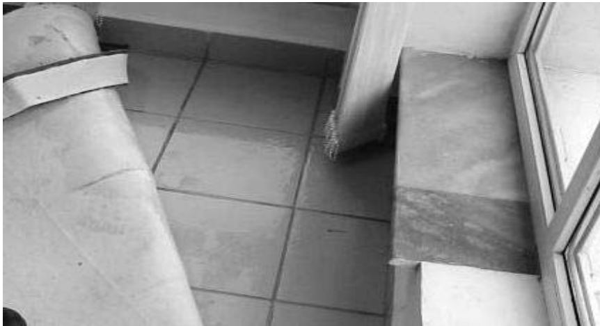
Fig. 7. Condensation on the floor made of sandstone [19]
