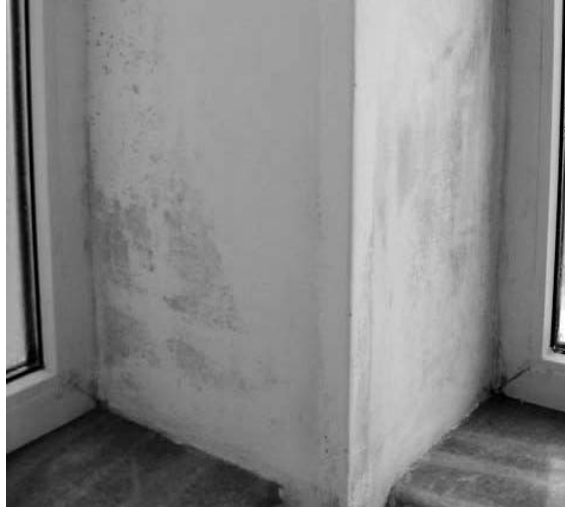
Fig. 5 Condensation at the corner pole
